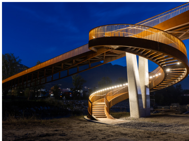
LaneLED WALL, Passerelle de Torretta Bellinzona
